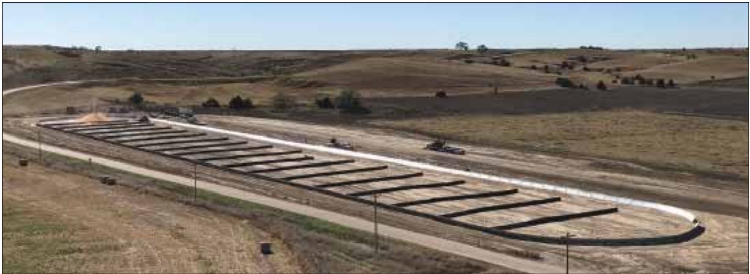
Frenchman Valley Farmers Cooperative's 2-million-bushel temporary storage bunker at Palisade, NE, which features unique perforated steel 4-foot-tall wall sections. Aerial drone photo by Frenchman Valley Farmers Cooperative.
