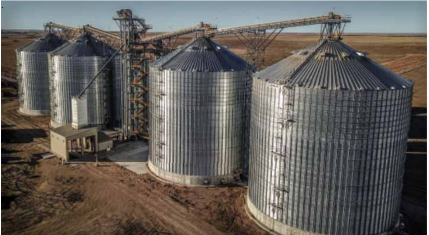
Dakota Mill & Grain's new 4.9-million-bushel rail terminal near Presho, SD. Drone photo courtesy of LandMarc Construction Inc.
