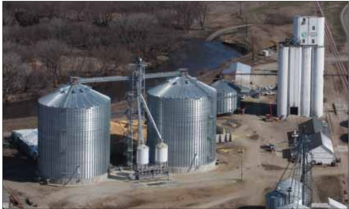
Aerial view of Central Valley Ag's branch elevator in Akron, IA, with a new 1.2-million-bushel steel annex featured prominently. Photos by JH Photography, Spencer, IA.
